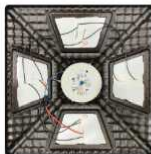
Inside Roof View
